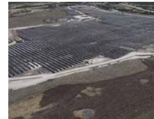
GES 3 Gaziantep SPP (Installed Capacity MWp 65)
