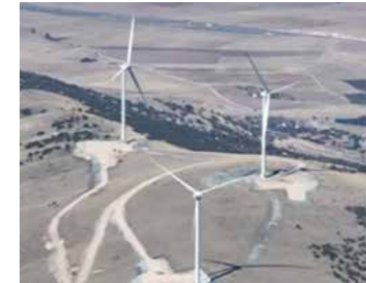
RES 3-Ankara-2-1 WPP (Installed Capacity MWe 50)
