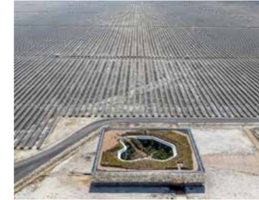
Karapınar YEKA-1 SPP (Installed Capacity MWp 1,350)
