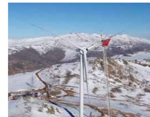
RES 3-Bayburt-5 WPP (Installed Capacity MWe 40)
